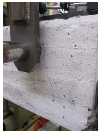
Figure 5. Photo taken before testing, at the end where failure later took place. Second test specimen, low corrosion
