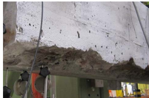
Figure 6. Photo taken before testing, at the end where failure later took place. Third test specimen, high corrosion with cover spalling.
