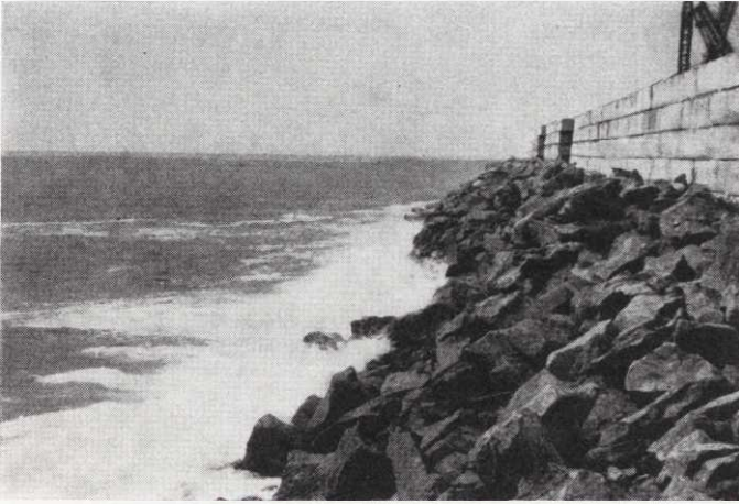
Fig. 12.3. The seaside of the rock-fill breakwater at Sinoe in Liberia. (Sinoe Dec. 1956)
