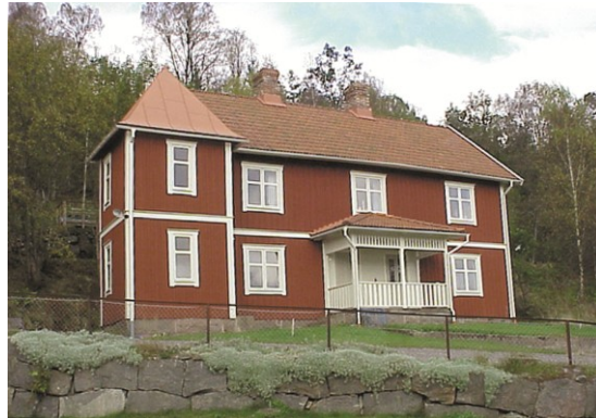
Figure 3. Tyreshill's façade, towards Southeast. Photo Eva Gustafsson, Heritage Halland at the Regional Museum Halland.
