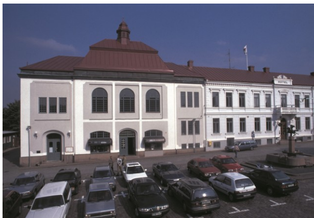
Figure 2. The South façade of Teatern, facing Hästtorget in Laholm. Photo Eva Gustafsson, Heritage Halland at the Regional Museum Halland.
