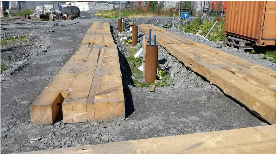
Figure A.4: *Steel extension pile and timber mat on top of fill material.*
