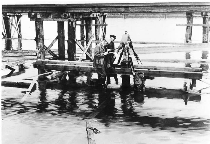
Figure 2.16: *Pile testing at Gothenburg's harbour circa 1910 using E. Wendel load frame (SGF Väst).*
