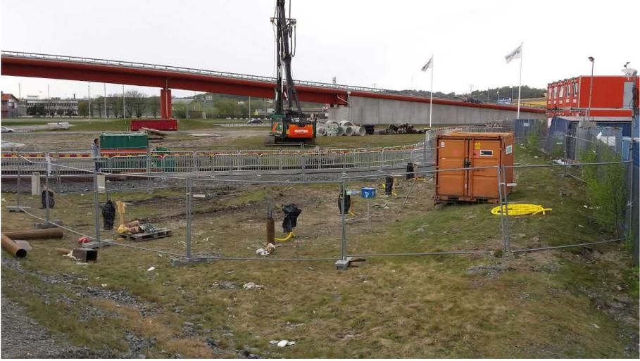
Figure A.3: *Test site after installation of the 6 test piles.*
