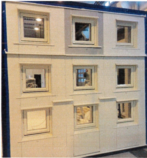
Fig. 2 Front façade of wall 1
