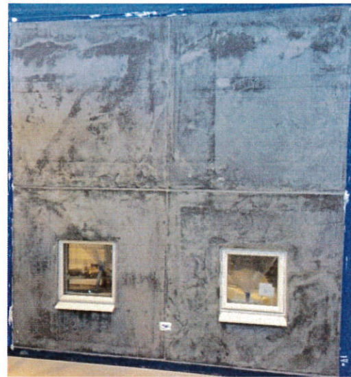
Fig. 3 Front façade of wall 2
