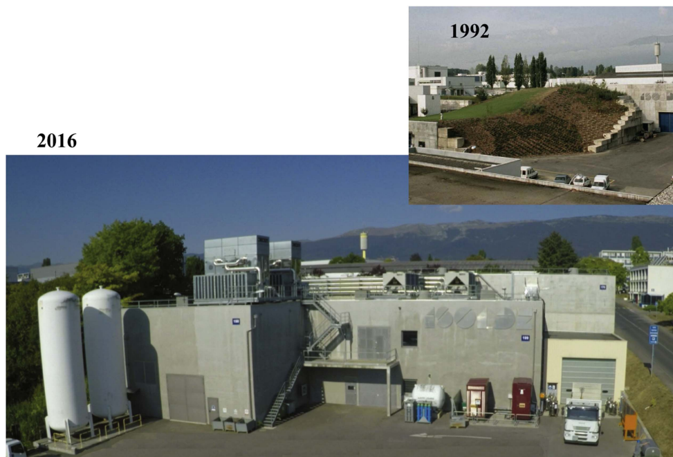
Figure 1. The upper photo shows the new ISOLDE building as it was in 1992. In this camera angle the photo is to some extent dominated by the target area. The protecting soil on its top became a small forest in the following years. The large picture from 2016 is totally dominated by the cryogenic installations for HIE-ISOLDE with two huge liquid He dewars in front of the target-area forest to the left.
