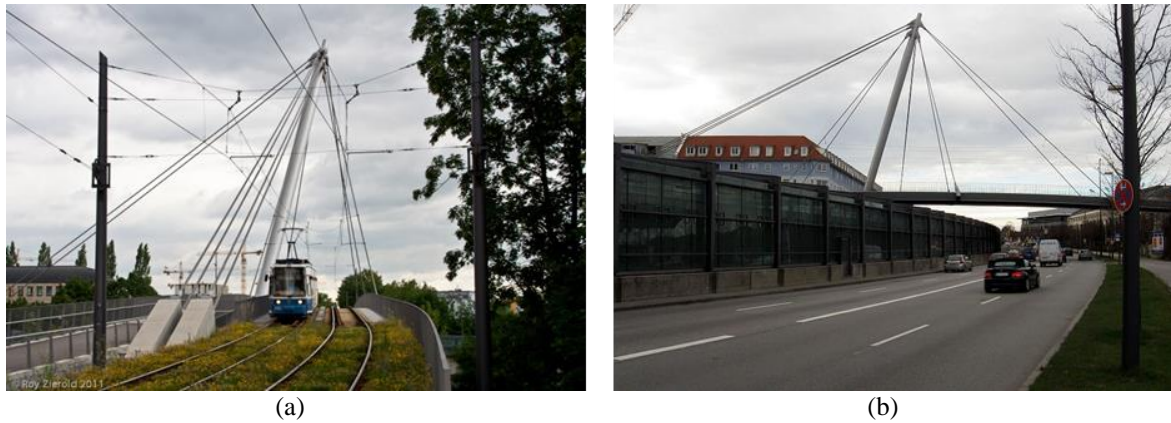
Fig. 2: Schenkendorfstrasse Bridge (Munich) from southern end (a) [17], and from east (b) [18].
