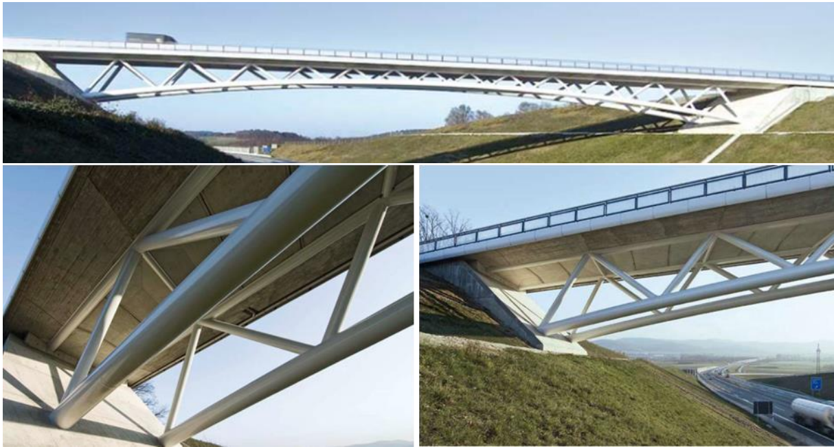
Fig. 4: Bridge over A73 Autobahn between Suhl and Lichtendels (Germany) [7].
