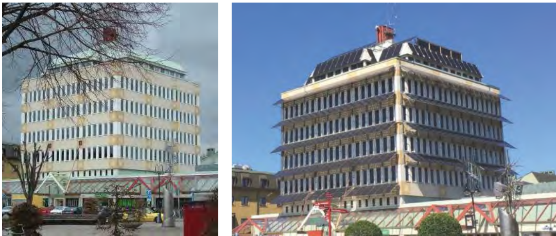
Figure 1: Alvesta Town Hall before and after addition of solar shading.
