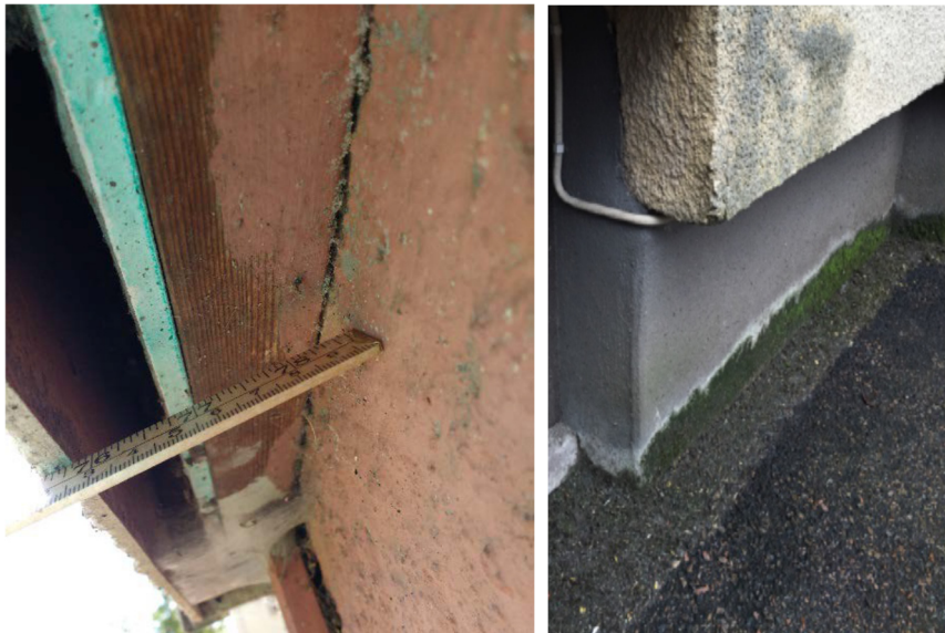
Figure 8. Example of two façades with additional insulation, seen from below.
