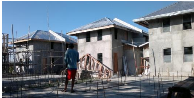
Pictures 5-7. Construction of ten two-story duplex houses, Iloilo City, March 2015 [11]
