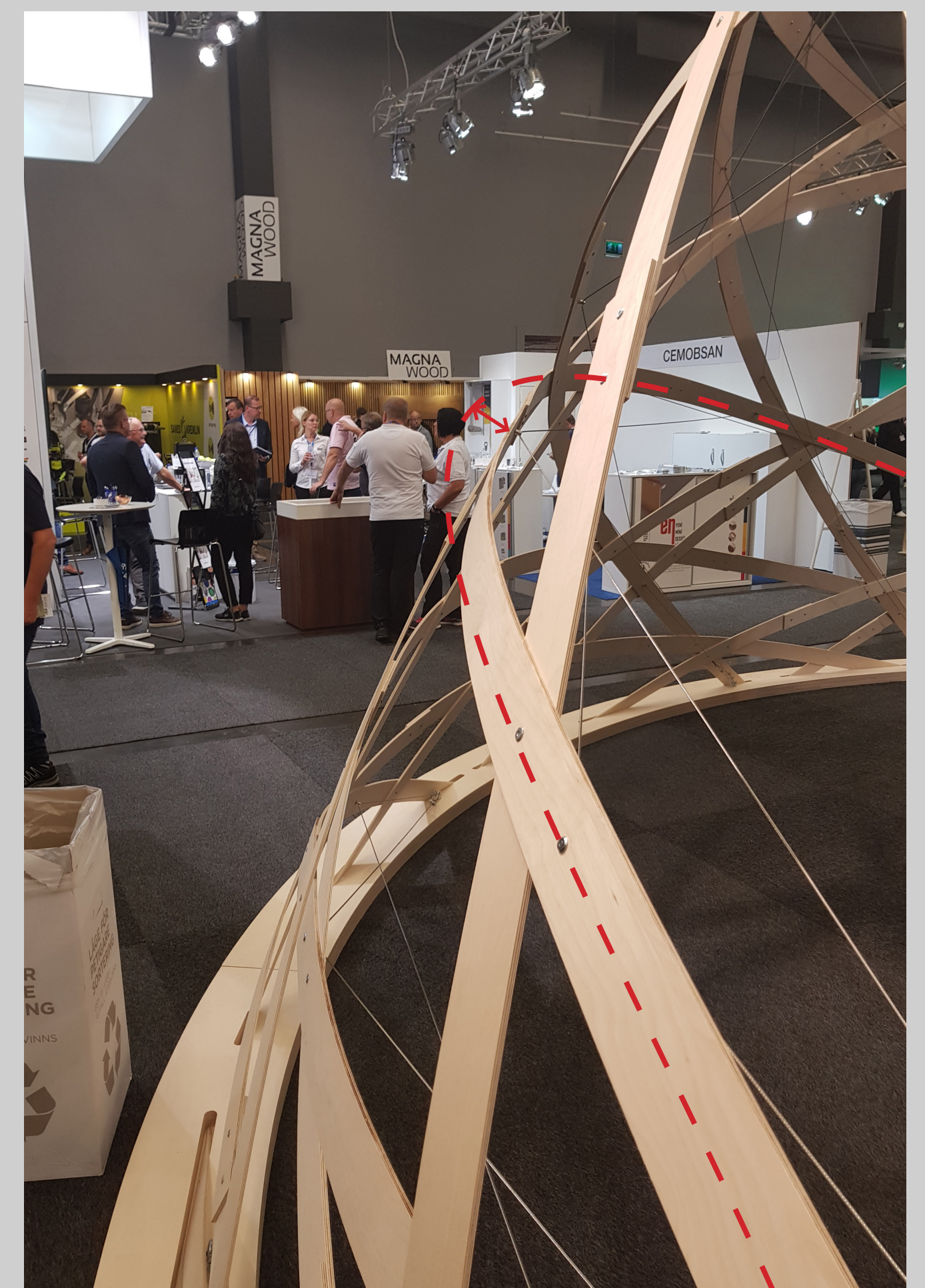
Figure 5: Lath curvature effected by pre-stress.
