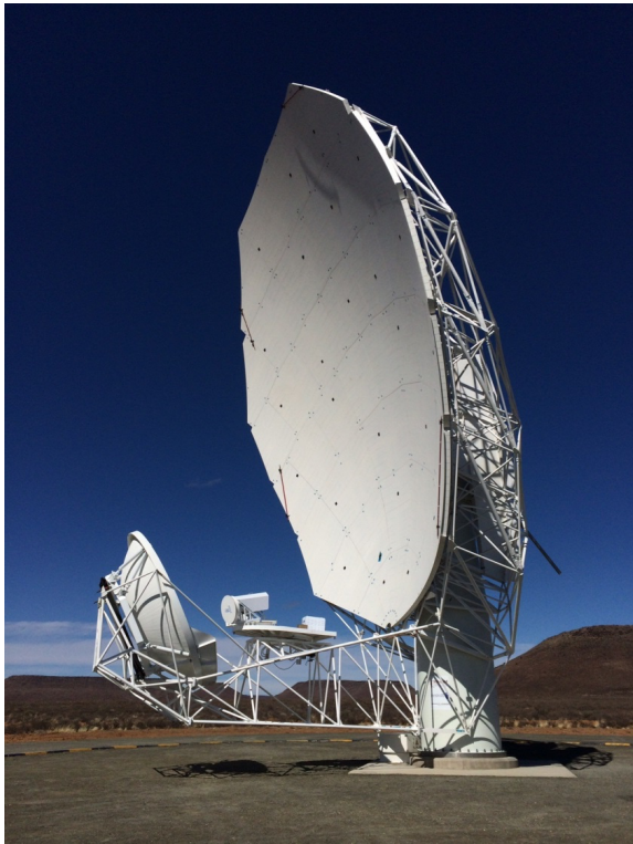
Fig. 1 Offset Gregorian shaped optics antenna proposed for SKA and ngVLA and used on the Meerkat array (unshaped, but as shown above. Note the large, easy access, platform for access to receivers.
