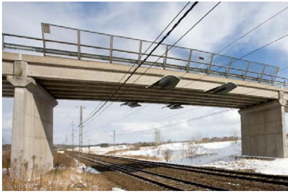
Figure 2: Concrete beam bridge investigated (source: NCC).
