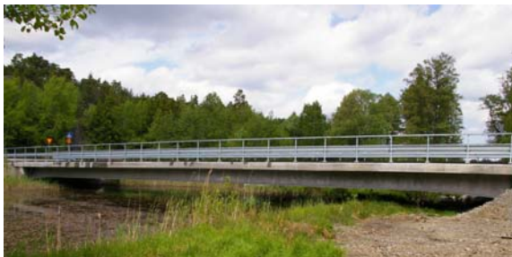
Figure 3: Steel-concrete composite bridge investigated (source: NCC).
