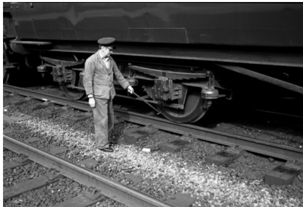
Figure 2.1: Wheel-tapper monitoring train wheels with the use of acoustics
