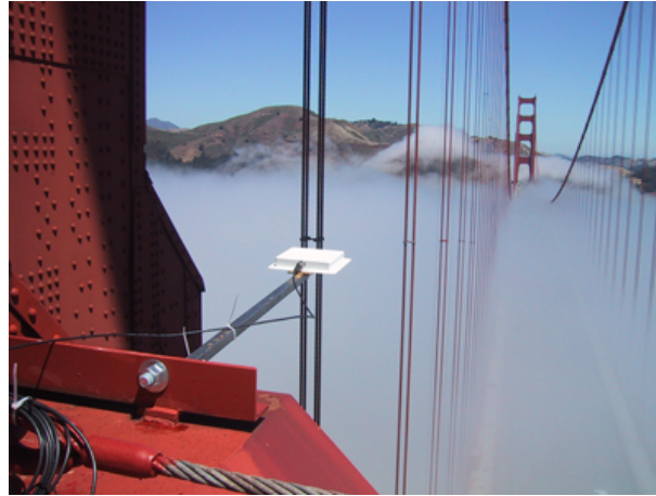
Figure 2.2: Accelerometer antenna sensor at the top of Golden Gate bridge (credit: Steven D. Glaser and Tommi Parkkila, ERCIM News).
