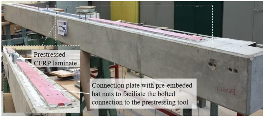
Figure 6. Self-anchored prestressed CFRP laminate on the RC beam after removing the prestressing tool and temporary anchors
