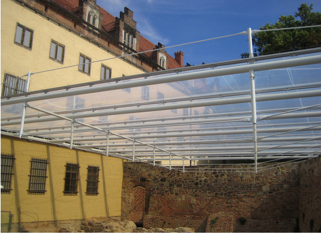
Figure 2.16: Lutherhaus, Germany (2010). Pressurised transparent foil cushions supported by cable supported steel beams.
