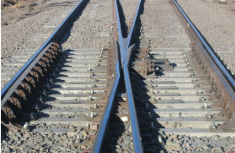
Figure 2.2: Overview of crossing panel from the front of the turnout including a fixed crossing and check rails. Photo provided by voestalpine VAE GmbH
