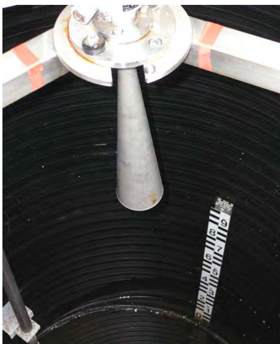
Fig. 2: The down-looking radar sensor, Campbell CS476, operating at 26 GHz, mounted at the top in the centre of the well.
