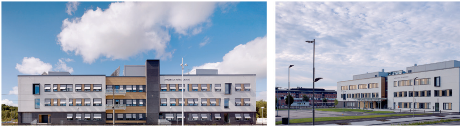
Figure 10. Photos Angered's Närsjukhus outside (photo by: Bert Leandersson)
