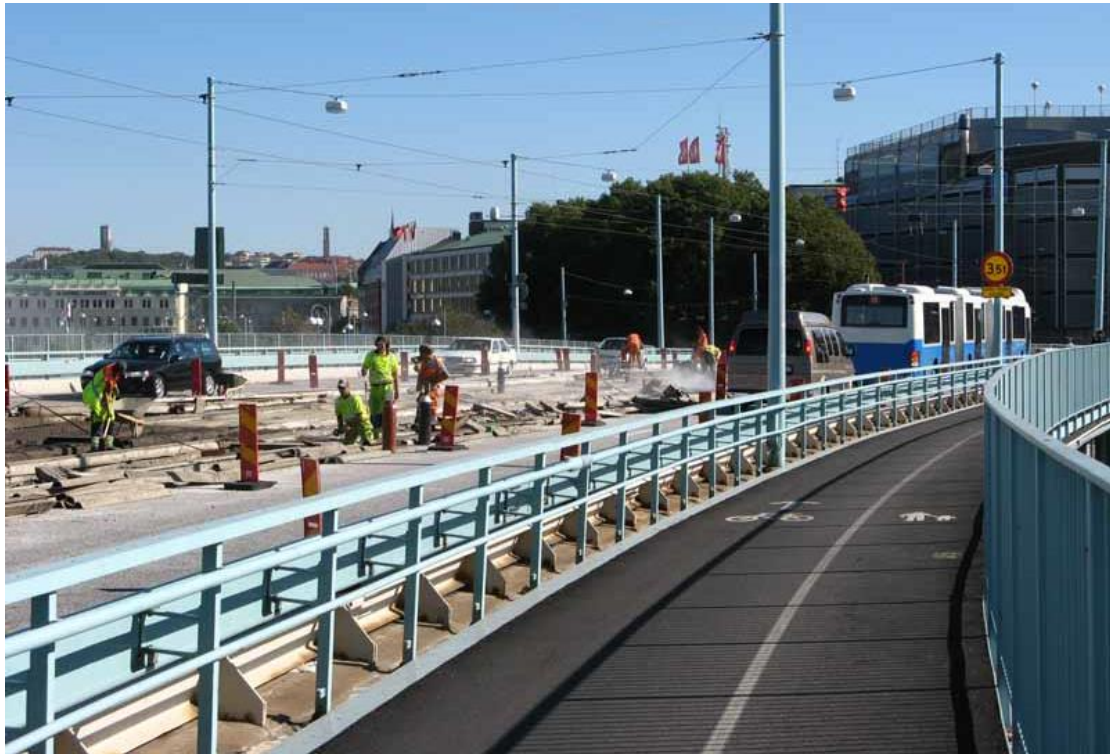
Figure 6. Götaälvsbron (after about 2 200 metres in the direction of figure 4b)
