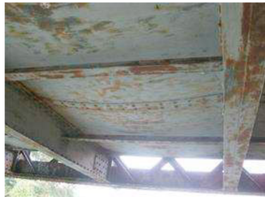
Figure 3 : steel-concrete composite deck (built around 1900)
