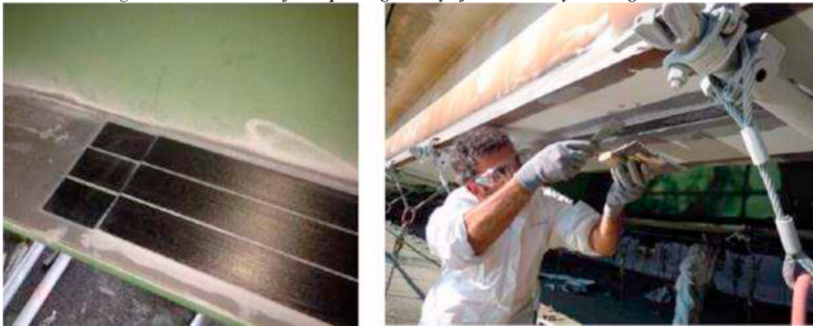
Figure 15 : Implementation of the carbon plates
