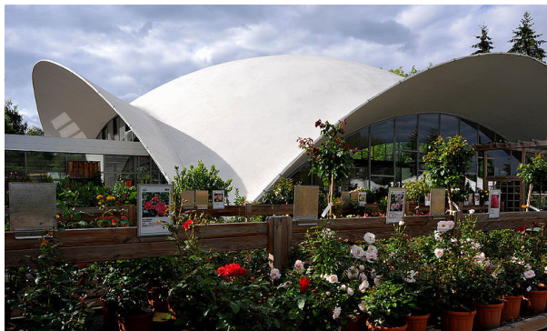
Figure 2-12 Concrete shell roof (Isler shell) of the garden centre Wyss in Zuchwil, built 1962; Solothurn, Switzerland.
