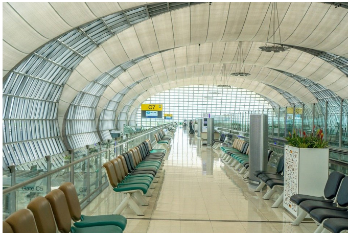
Figure 2-17 The structure of the terminals at Suvarnabhumi, Bangkok international airport, uses textiles in a multiple layer system.
