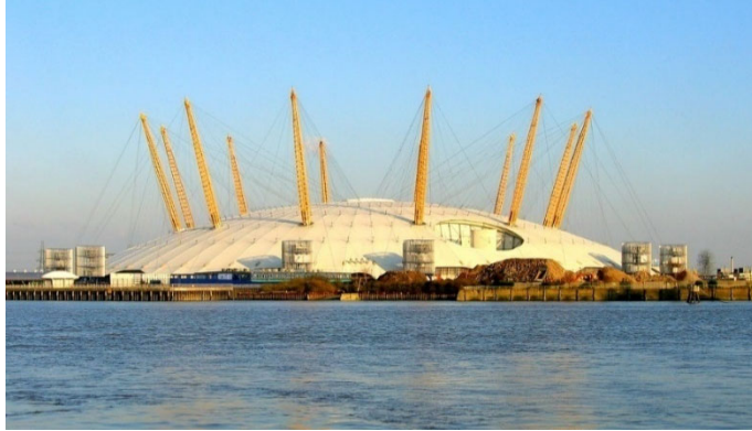
Figure 2-16 Millennium dome (O2 Arena), in London. A large textile dome.
