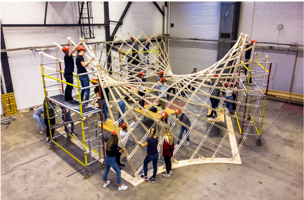
Figure 2.29: Asymptotic grid shell under construction, built with students in the course Parametric Design - Digital Tools with bachelor students at the Architecture and Engineering program in 2019. The author was the part of the design team together with I. Näslund, J. Isaksson, H. Moubarak and C. J. K. Williams
