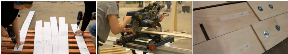
Figure 7: Fabrication of the laths using paper templates a) drilling holes for the slots and the joints. A paper template was printed aid this process b) The slots were finished using a pre-calibrated chop saw, cutting halfway through the width of the lath c) The laths were assembled into full length using two m6 bolts and nuts.
