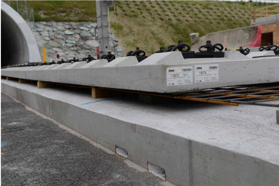
Figure 2.4: The STA system during construction. Note that the asphalt used as a base layer for the track in the photo is normally not used by STA. From STA [5].
