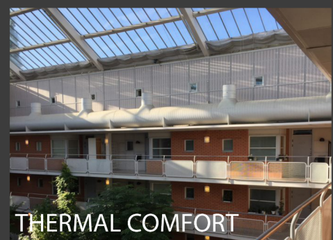
Höstvetet, Stockholm - solar shading prevents over temperature caused by high solar load
