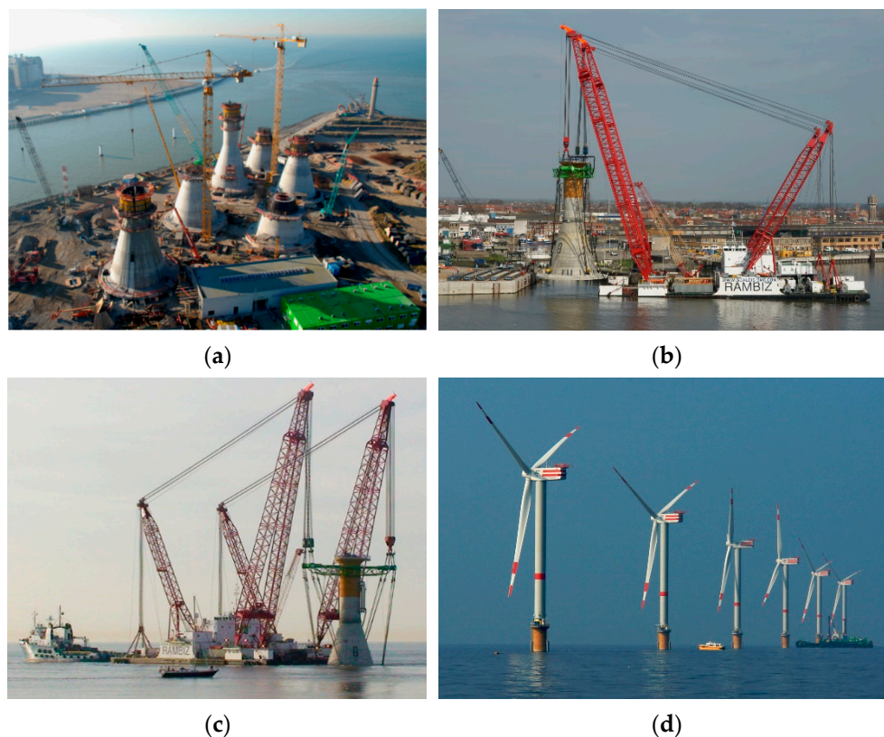
Figure 8. Construction and installation of gravity-based substructures for Thornton Bank wind farm: (a) construction yard by the access channel to the port of Ostend, Belgium, (b) load-out operation, (c) transport and installation and (d) after turbines installation. Credit: C-Power NV, reproduced with permission.
