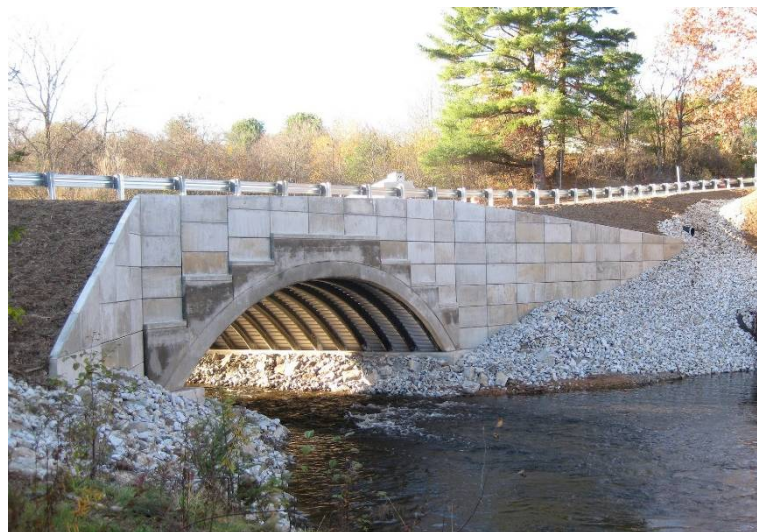
Figure 2. Royal River Bridge in Auburn (USA) with a span of 11.6 m, composed of 13 concrete-filled FRP curved tubes [20].
