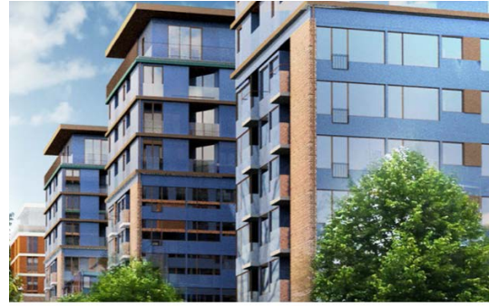
Figure 2. A 1960s building where the original teak windows were allowed to be replaced by new ones. Photo: Private company
