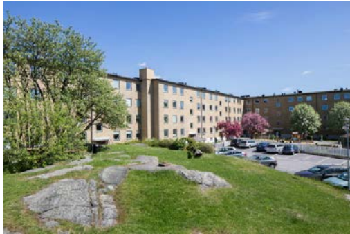
Figure 1. A residential area with replaced brick facing the courtyard and new board material on the more exposed outside facades. Photo: Private company
