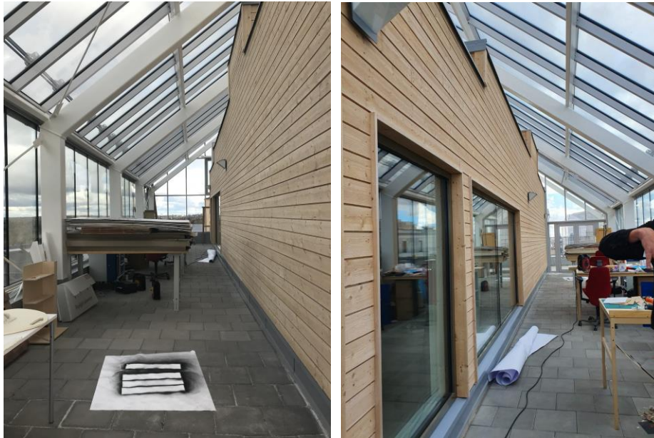
Figure 4.19. Study places in the unheated part of the rooftop.
