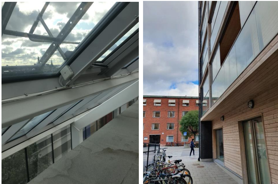
Figure 4.20. There were some problems with rain leakage around windows (left), glazed balconies (right).
