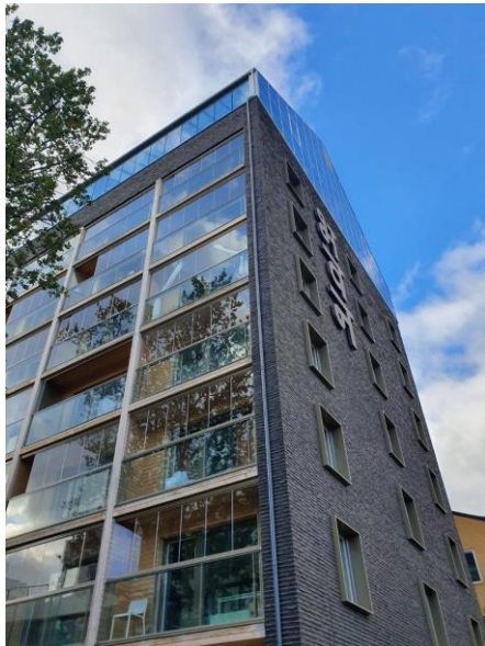
Figure 4.18 KTH Hemmet showing the glazed balconies and glazed rooftop.
