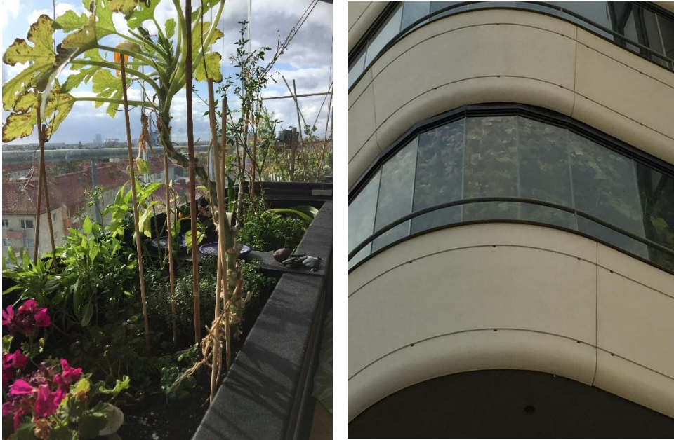
Figure 5.3. Glazed balcony with room for farming.
