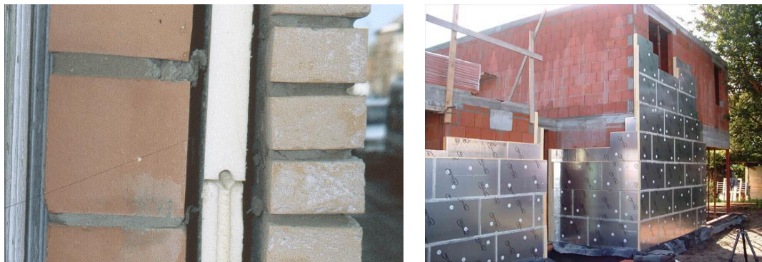
Figure 2: Installing cavity wall insulation: poor (left) versus good (right) workmanship
