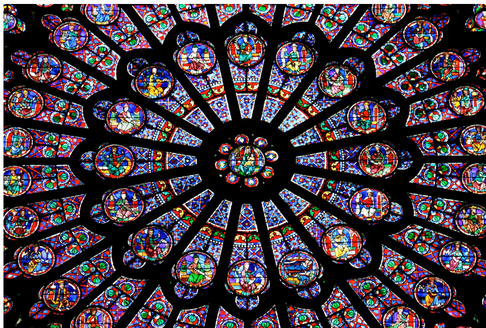
Figure 4.5: Medieval application of localized surface plasmon resonance. Light in certain wavelength intervals is absorbed and scattered by metal nanoparticles in the glass, producing colorful results. Notre-Dame de Paris.
