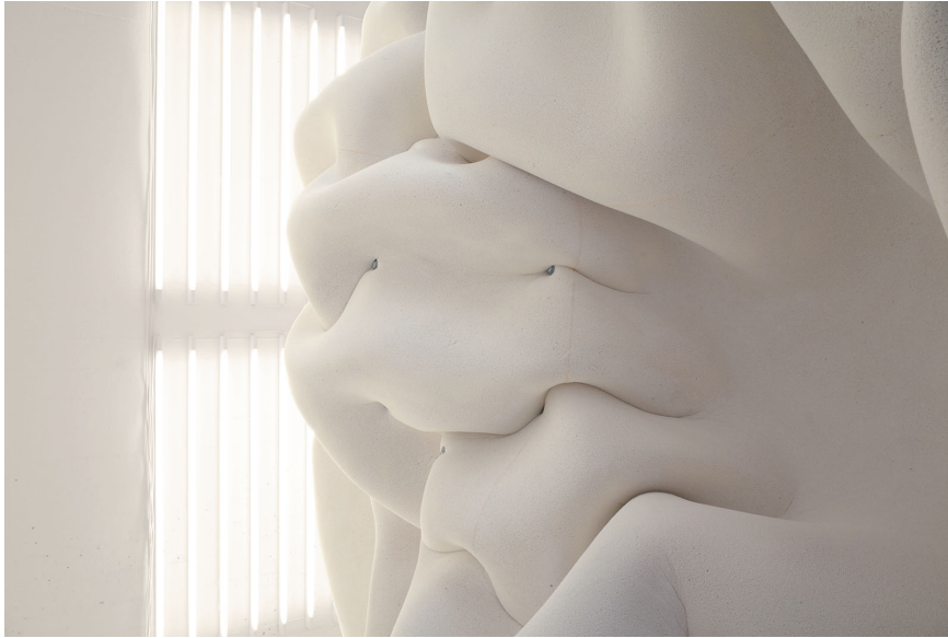
Figure 3.8. Erratic , Aalto University Digital Design Laboratory, 2013. Installation detail showing constrained polyurethane surface finished with plaster powder.
