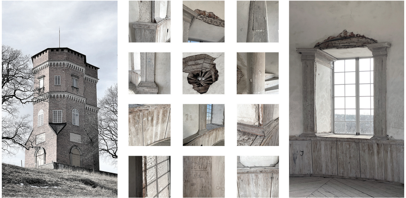
3 Eighteenth-century tower 'Götiska tornet' in Stockholm, Sweden (left), with an inventory of deteriorated wooden elements (middle) and an incomplete wooden window casing selected for the experimental restorative intervention (right).
