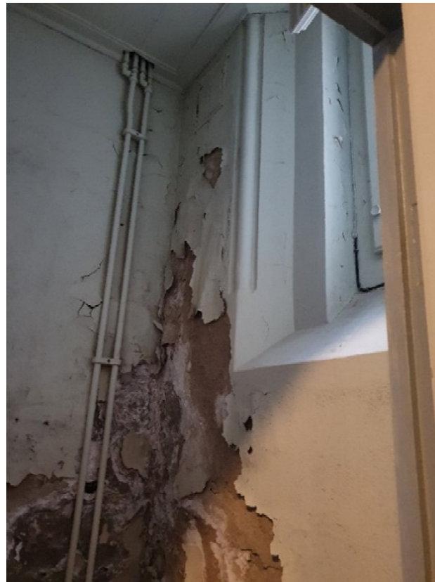
Figure 8. Example of the moisture-related damage at the interior of the Örgryte New Church: weathering of the internal coating mortar (plaster) and paint, and salt efflorescence. Photo: the authors.
