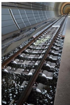
Figure 4. Sleepers adapted for two auxiliary rails in a transition zone between a ballasted track and a slab track inside a tunnel
