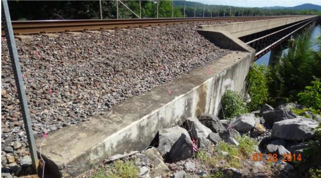
Figure 11. Bridge transition zone with concrete confinement wings walls parallel to the track.
