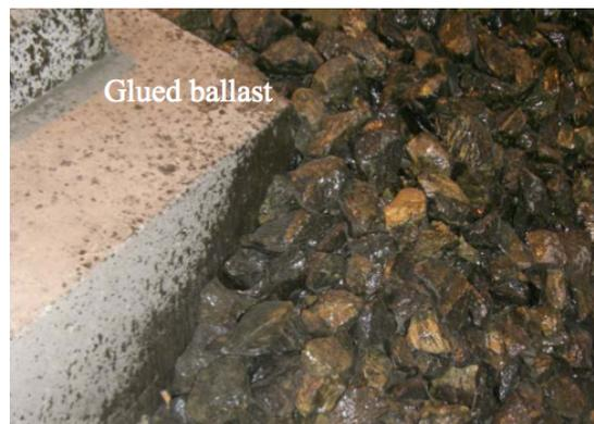
Figure 6. Glued ballast [55]
