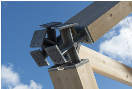
(b) Detail of the joint, Crossrail station Canary Wharf, London © Nigel Young/WIEHAG
