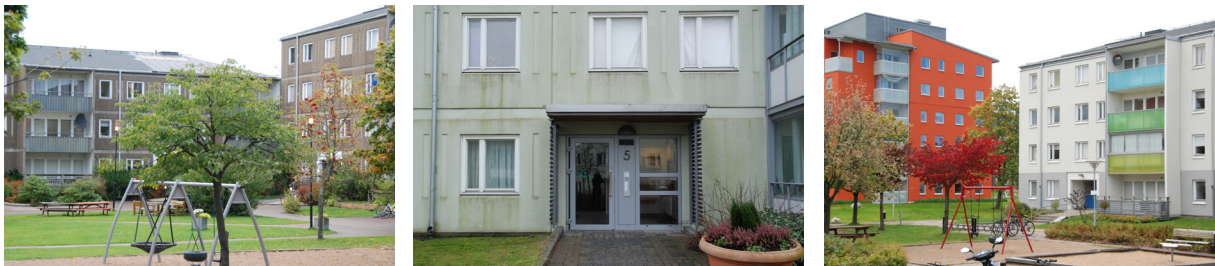
Figure 2 Case B before (left) with sea-stone facades and after (middle) renovation of phase two. The sea-stone façade was painted pale green to make it more attractive, a solution that has not aged well. To the right, the red pilot project with high energy saving and the coloured balconies from a recent phase of the renovation.
