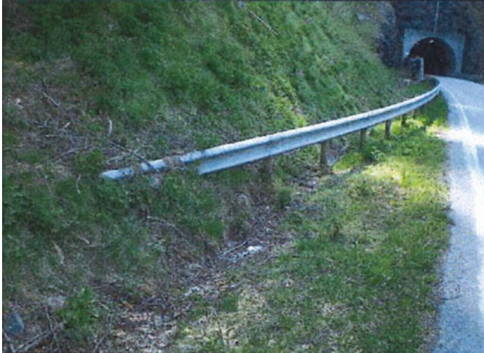
Fig. 5 Flared out guardrail terminal attached to backslope. (Photo: Marianne Gjerde (2008))
