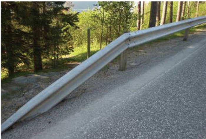
Fig. 4 Turned down guardrail terminal. (Photo: Marianne Gjerde (2008))
