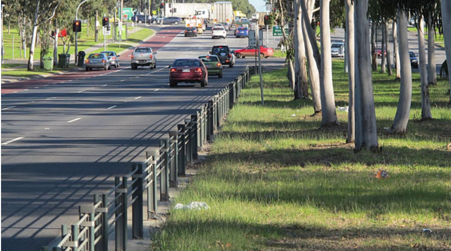
Fig. 16 Continuous flexible barrier systems to manage kinetic energy in lane departure crashes along high-speed, high-movement roads (Melbourne, Australia)
