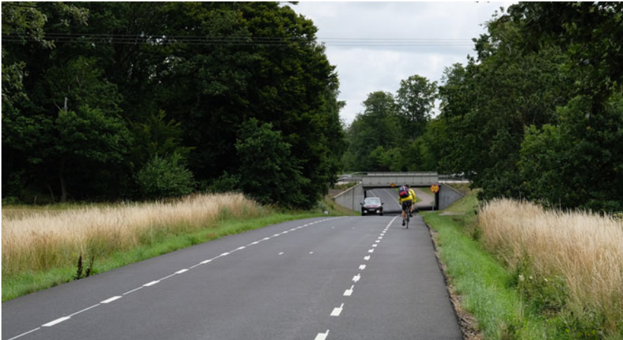
Fig. 5 Example of Two-minus-one-road from a Swedish pilot study. (Source: Visser van der Meulen and Berg 2018)
