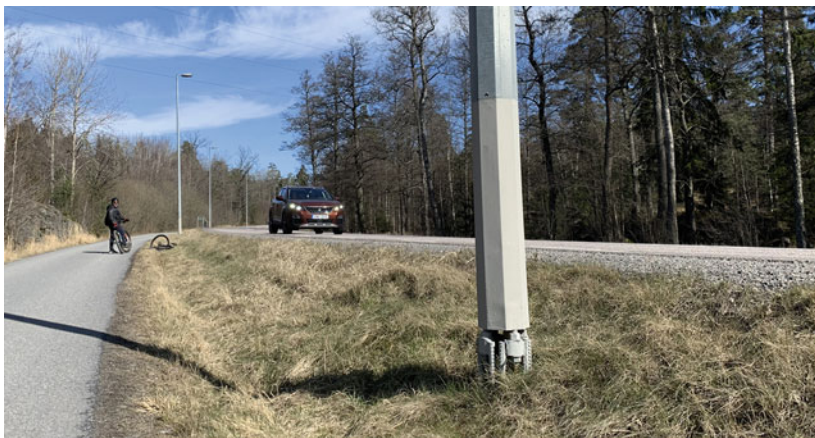
Fig. 16 Lightning column with a deformable element in the base aimed to lower vehicle acceleration in a crash. (Photo: Helena Stigson)
