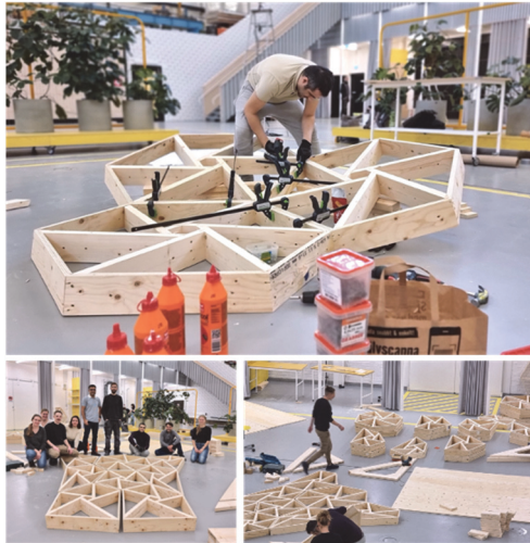
Figure 14 Easy and rapid assembly of the polygonal cassettes
