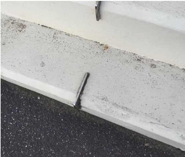
Picture 2 Skate stoppers installed to prevent skateboarders from grinding on the steps in Melbourne, Australia
