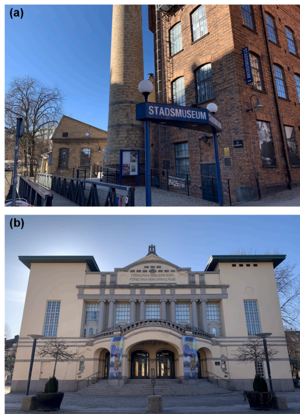
Fig. 4. A case study was conducted in two public historic buildings: (a) the City Museum and (b) the City Theatre in Norrköping, Sweden.
