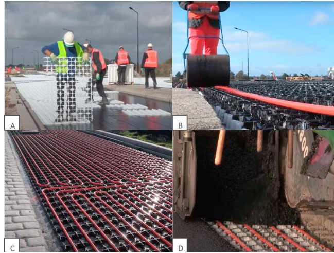
Fig. 5. Using plastic mesh for positioning the pipe. (www.ooms.nl)
