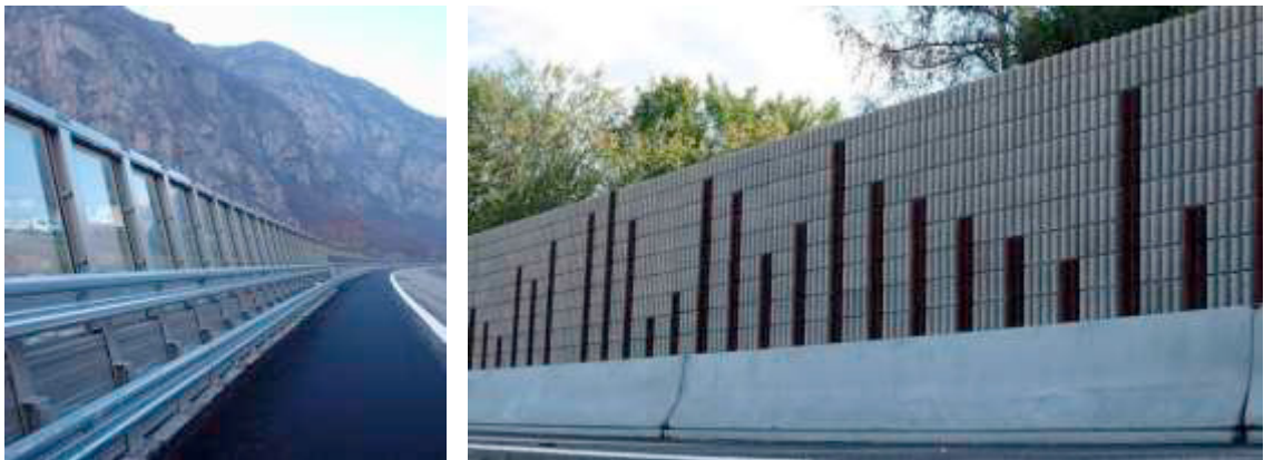
Fig. 2. Different types of integrated noise and safety barriers of different materials in Europe (steel & transparent left side and fully concrete type right side).
