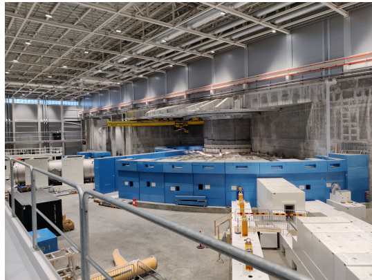
(c) ESS (under construction)
