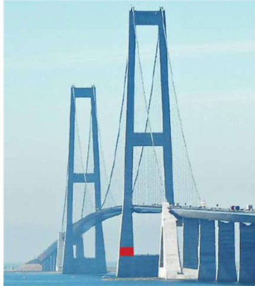
Figure 1 Automatic Sniffer measurements at the Great Belt bridge are conducted from the eastern Pylon (marked in red). Here 25000 ships are passing annually to reach or leave the Baltic Sea. Chalmers has measured more than 20,000 ships at this site since 2015 (Mellqvist 2018).
