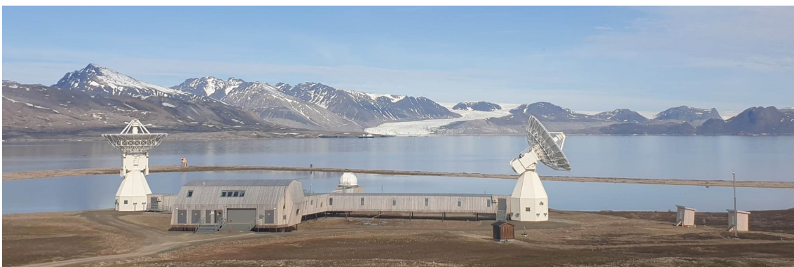
(b) The new telescopes NYALE13N (VGOS equipment), left, and NYALE13S (S/X equipment), right.
