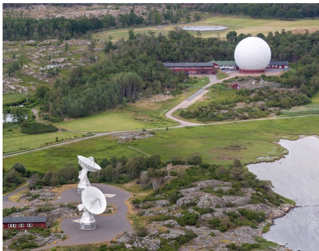
Figure 4.1: Radio telescopes at OSO used for ONTIEs: the legacy S/X telescope ONSALA60 (radome, top right corner) and the VGOS twin telescopes ONSA13NE and ONSA13SW 2 .
