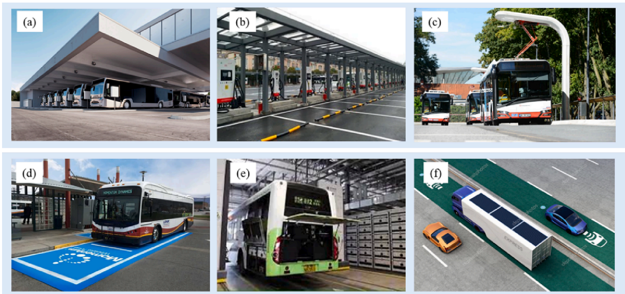
Fig. 1. Typical e-bus charging infrastructures. (a) Terminal charging station allowing overnight parking and charging (ABB Group, 2021). (b) Depot charging station with plug-in chargers (Co, 2021). (c) Opportunity charging station equipped with pantograph chargers (Lehmann, 2021). (d) Opportunity charging station with a stationary wireless charging pad (Lambert, 2018). (e) Battery swapping station (XJ Group Corporation, 2021). (f) Dynamic wireless charging lane (Chesky, 2021).
